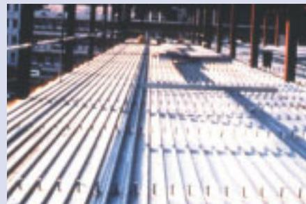
**Composite construction using steel decking**
