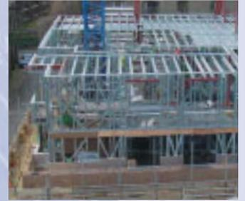
8-storey light steel Metframe construction. This minimises the load on the underlying Brunel railway tunnel, Rotherhithe.
