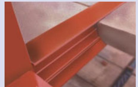
**Slimflor beams supporting precast concrete slabs**
