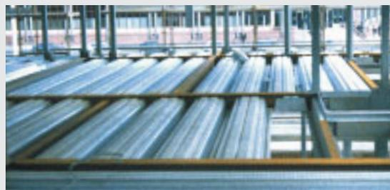
*Slimdek*<sup>®</sup> eliminates the need for downstand beams
