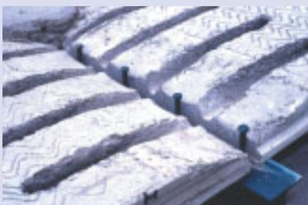
**Steel beams supporting precast concrete slabs**
