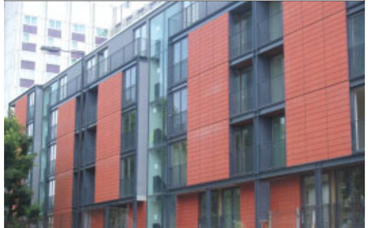
A 6-storey mixed modular and light steel structure has been constructed at Lillie Road, Fulham for the Peabody Trust, by Forge Llewellyn. It consists of 40 prefabricated light steel floor and bathroom modules, together with a tubular steel structure to provide stability.
